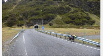
Entrance of the notorious North Cape Tunnel. Are the stories exaggerated, or was I lucky? [32]
